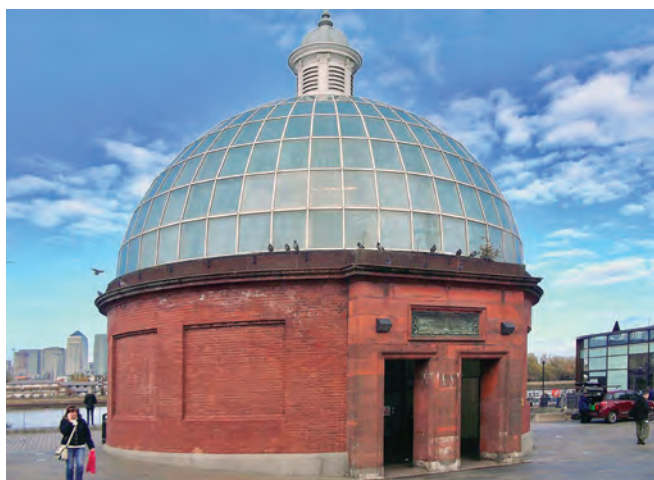
Greenwich foot tunnel south entrance
